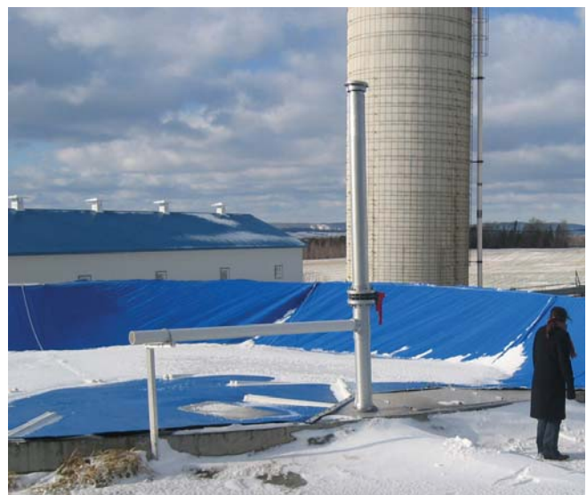
Negative air pressure covered manure storage
