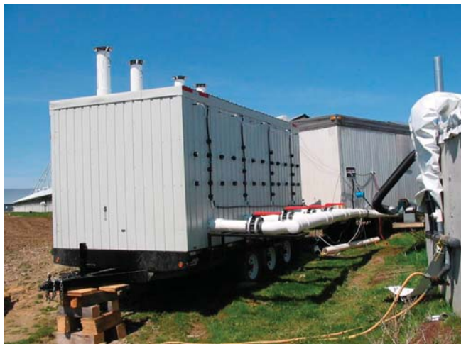
Large-scale experimental biofilter operating on a covered manure storage
